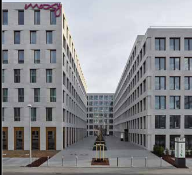
Quartier West | Darmstadt, Germany
